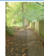
Logs Path Uneven, narrow footway
