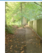
Logs Path Uneven, narrow footway
