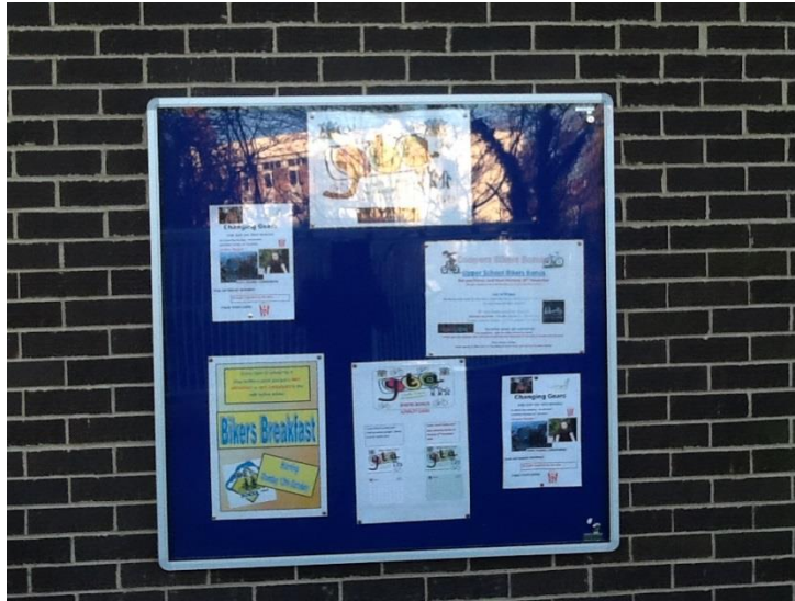
External Notice Board by Bike Sheds
