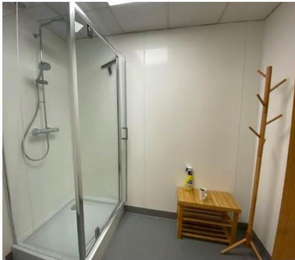
A second shower room has now been installed, including a bench and mirror.
